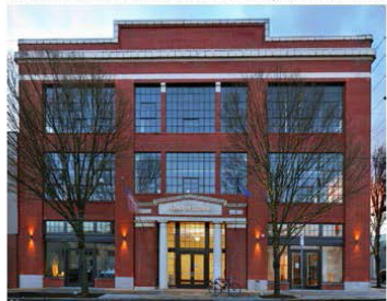
Replacement windows on the ground floor restore the historical character of the building. Photo by Sally Painter. (SE Division St and 10th Ave)
