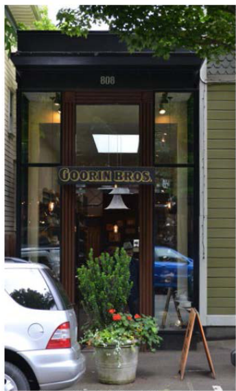
Narrow building maximizes day lighting with transom windows and a skylight (NW 23rd Ave and Johnson St)
