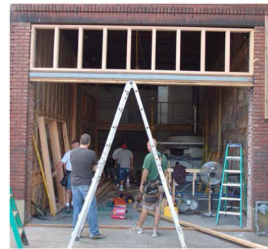
Contractors replacing a storefront with durable wood windows.
