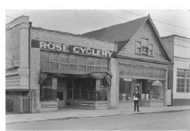
Historic photo from 1929 shows the benefits of retractable awnings and transom windows on a grey Oregon day.
