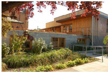
Martha H. Terrell Community Services Center uses a green roof, living screen wall & large storm planters to make a rich environment. (NE Alberta St and 8th Ave)
