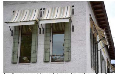
Operable awnings and shutters control how much sunlight enters the building (NW 23rd Ave and Flanders St)
